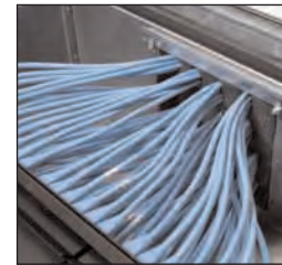
Firestop block adds protection to network wiring
